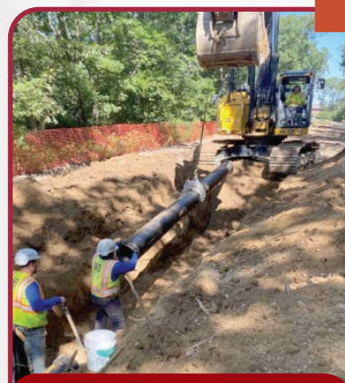
Ongoing infrastructure improvements strengthen BWD's water distribution system.
