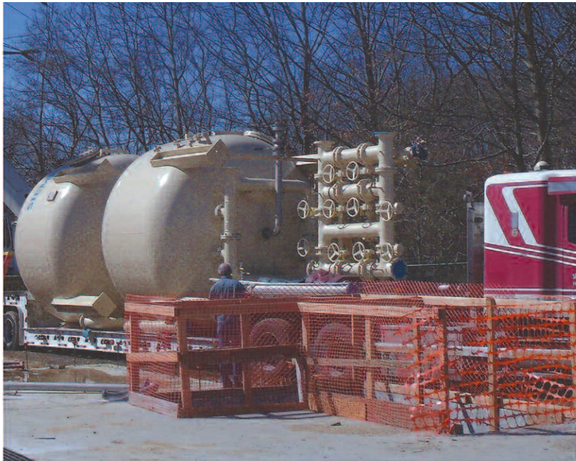
Carbon filters being lowered into the ground at Plant 4.
