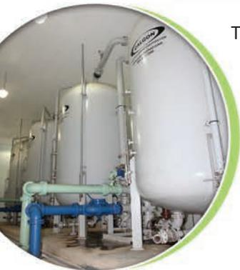
The District is happy to report that this facility is currently online with four GAC filters that are fully operational to ensure the delivery of the highest quality water for our customers. In the Spring, the District will be rehabilitating the two additional buildings on-site with a new roof and siding.
